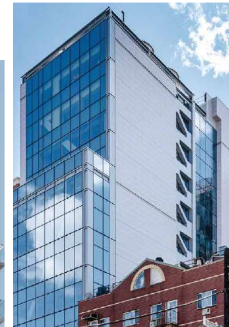
The monochromatic cladding of the ventilated porcelain façade is made up of large-format pieces of three models: Ferroker Niquel, Extreme White by STON-KER® and Deep Light by Solidker. The side wall in Ferroker Niquel porcelain stands out against the existing brick building. Photos: Imagen Subliminal
